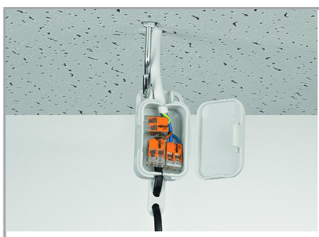
Pendant light connection in suspended ceilings
